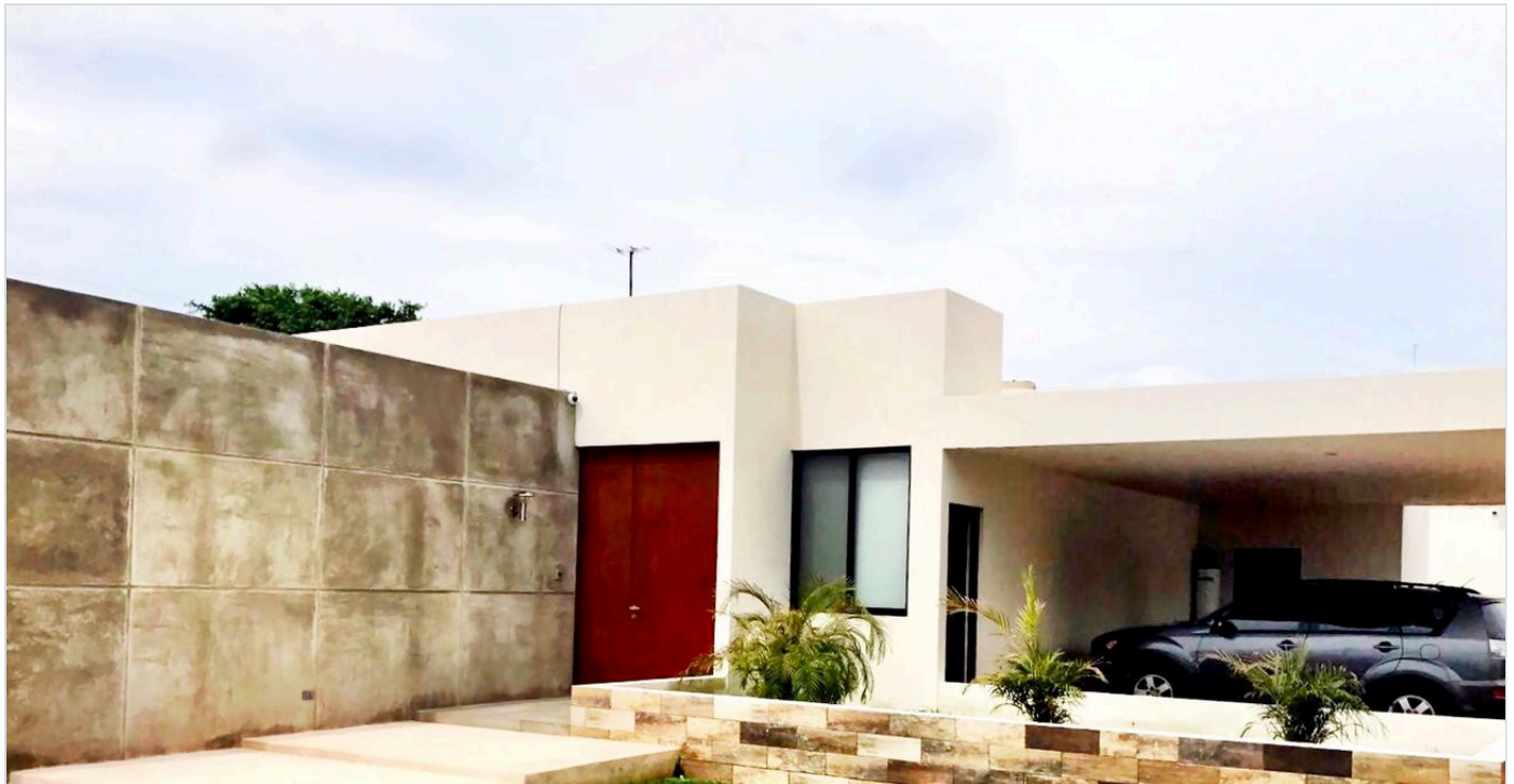
Fig. 7 A finished Urbex home.
